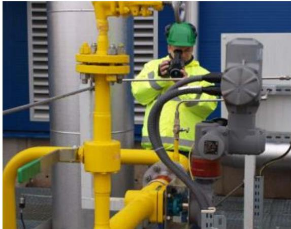
Figure 2 Localization of gas leaks
